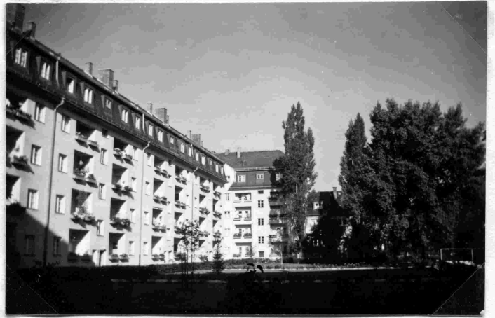
View from rear of Frau Walter's; the building dates to approximately '30.
